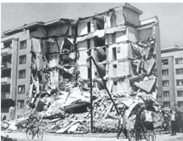
Figure 1. Destroyed residential masonry building (five storeys) [3]
